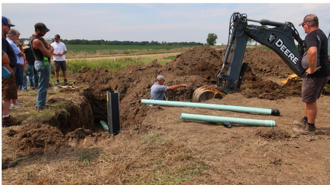
Participants at the drainage water field day watch as the tile plow begins to dig in new pipe as part of a saturated buffer installation demonstration. Photo credit: Ehsan Ghane
